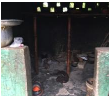
Not acceptable: Kitchen with insufficient ventilation
