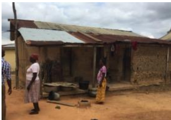
Not acceptable: Mudbrick walls in poor condition
