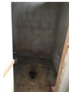
Acceptable: Pit latrine with concrete slab
