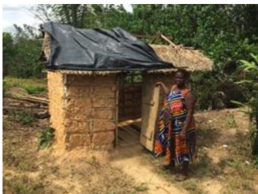
Not acceptable: Pit latrine with wooden slats
